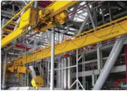
Ex-Proof Wire Hoist (Low head type Monorail)
